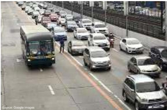
**BUS AND PUJ LANE LINE** – a solid yellow line used to separate other vehicles from buses and PUJs and supplemented by raised pavement markers
